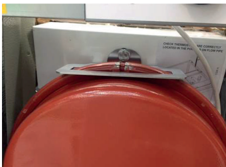
Figure 7-5: Vessel fitted on cleaning door
