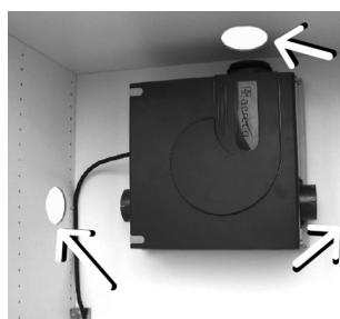
17. Carry out the holes for the passage of the ducts in front of the inlet and outlet sleeves.
