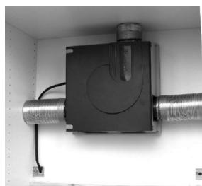
20. Connect the 2 extract units and the extract grille: the fan is ready to operate !
