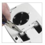
Lubricate the supply pipe ends using a silicone based lubricant and carefully slide the Aquastream Thermo unit onto the pipes whilst feeding the low voltage cable through the cable entry point. Secure the unit to the wall using the screws provided.
