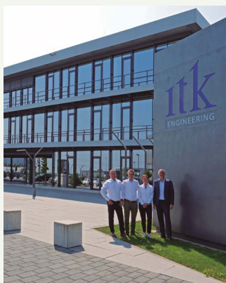
ITK Engineering GmbH. An innovative office building located in Germany. ECOi - PACi
