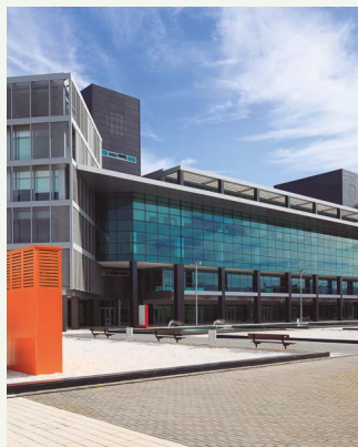
Andalusia Technology Park. Offices of high energetic efficiency. Spain. ECOi
