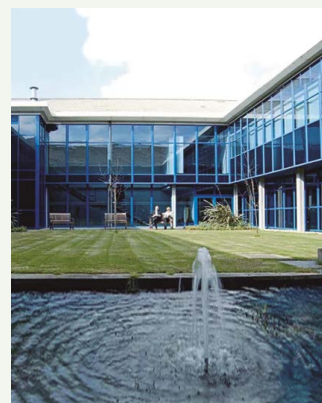
NHS Canford house clinic, Bournemouth, UK. VRF
